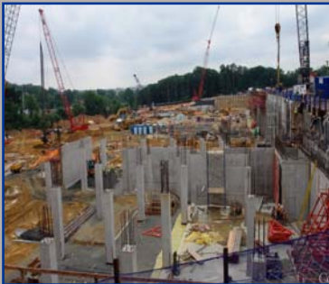
Mark Center Office Park 1.7 Million SF Under Construction
