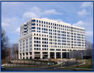
7930 Jones Branch Dr Delivered 323,698 sf in Tysons Corner
