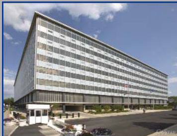
2100 2nd Street, SW U.S. Coast Guard Renewed for 592,000 SF
