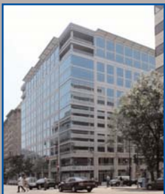
The Executive Building Delivered April, 2008 332,000 SF Available for Lease
