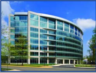
3120 Fairview Park Drive Delivered 183,353 sf in Merrifield
